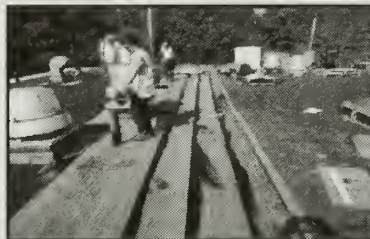
Two plies of a reinforced waterproof felt were installed in a cold applied asphaltic adhesive to the top of the insulation
